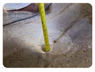
Fill hole with two-part epoxy to within 2 inches of the top of the hole.
