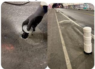
Measure the depth of the hole. Recommended depth is 4.25 inches.
