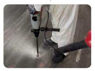
Blow out the hole. Clean road or walkway surface of dirt and dust. Please remember to wear safety glasses!
