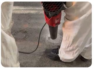
Place Heavy Hitter anchor with glue guard and supplied bolt in hole and firmly press and twist anchor against road surface. Make sure anchor stays against road surface.
