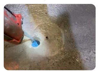
After epoxy is cured, install Heavy Hitter until firmly against road surface, then installation is complete. (Relton Cutter Head #SB-32 2" - Relton Shank #SMX-10 - Hilti HY 200-AV3)
