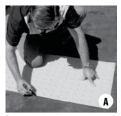
A. Using a broom or blower, remove dust and debris from area of installation. Align the DWT Smart-Tile in proper orientation on concrete surface. Outline the concrete surface around the DWT Smart-Tile using an ink marker and then remove tile.
