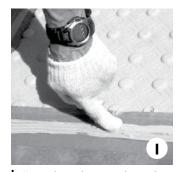
I. Use a plastic shaping tool, spatula or a gloved finger to shape the adhesive that has oozed from underneath the DWT Smart-Tile. Make a cupped shape profile between the tile edge and adjoining concrete.
