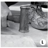
While still applying pressure to the tile, completely insert stainless steel anchor into molded dome recess and lightly hammer down pin with mallet. Installed stainless steel anchor should be flush to the top of molded dome. Be careful not to overdrive anchor.
