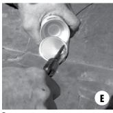
**E.** When using AdcoSeal Körapur 125 adhesive/sealant, be sure to remove peel-away protective cover on bottom of cartridge and remove desiccant prior to loading into caulking gun. Only use adhesive supplied by the manufacturer.
