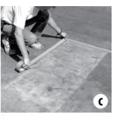
**C.** After grinding surface, remove dust or debris with a broom or blower. Place masking tape on concrete just outside inked lines (approximately ¼" from edge of tile).
