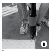
K. Allow adhesive to cure a minimum of 30 minutes prior to drilling holes for stainless steel anchors. While continuing to apply pressure to the DWT Smart-Tile, use a ¼" masonry drill bit and concrete drill, drill a 2" deep hole; blow dust from hole prior to installing stainless steel anchor.
