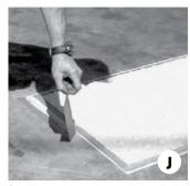
J. Immediately remove tape from the DWT Smart-Tile and concrete surface. Any adhesive on the DWT Smart-Tile surface can be removed with mineral spirits.
