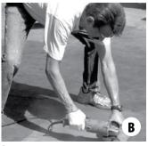
**B.** It is important to remove dirt, curing agents, topical color, oil, grease or other contaminants from the concrete surface by scouring the surface between the inked lines using a grinder with a wire cup attachment.
