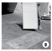
**D.** Place masking tape along outside perimeter of tile (about ¼" from edge) to protect the *DWT Smart-Tile* surface from excess adhesive oozing from under tile.
